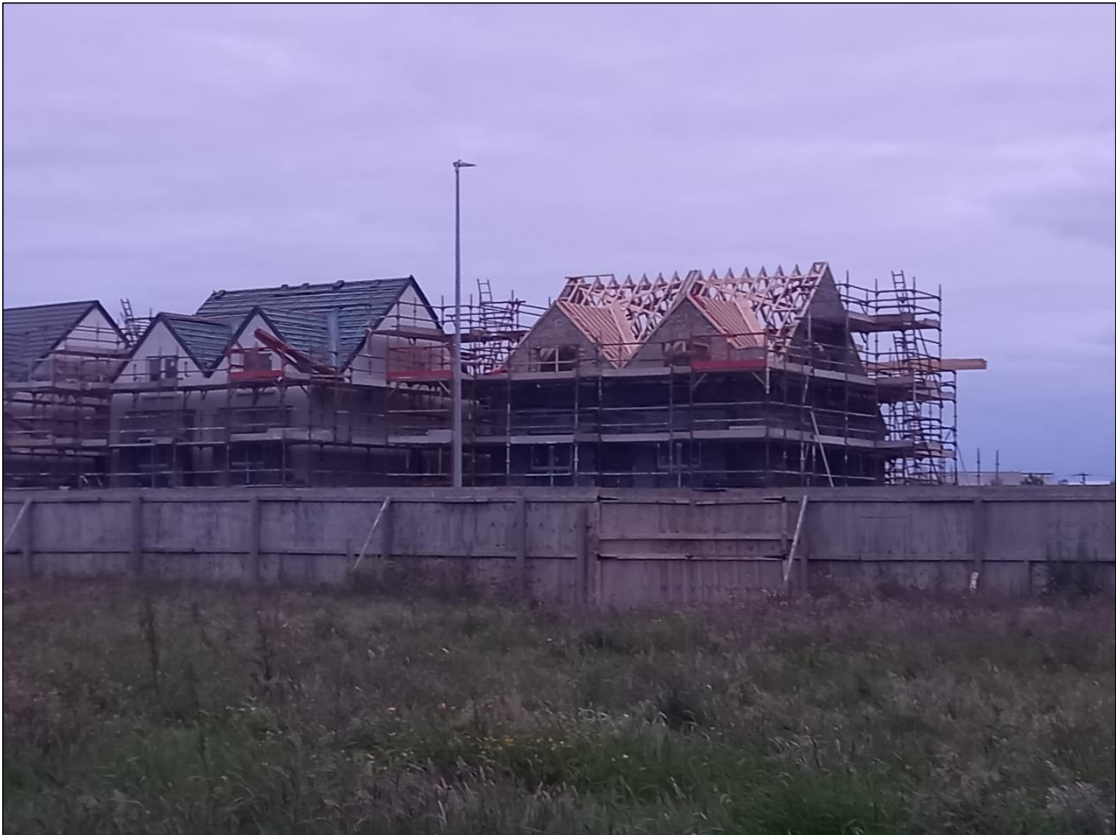
Plate 2-4 Hoarding present along the southern boundary of the proposed development site.
